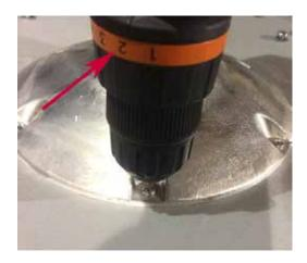
Attach the **k-plate** driving the **6 wood screws Ø4mmx12mm** (**#8x1/2"L**) into the table top **without over-tightening** (set your power-tool on **LOW TORQUE** if using a power tool). Screw size can be increased all the way up to Ø6 mm (1/4"Ø).
