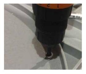
Using a 6mm allen key, drive the **inserts** into the table top holes made previously **without over-tightening** (set your powertool on **LOWER TORQUE** if using a power tool).
